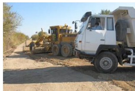
Construction of new road in Gengeshlik “Chovdur” in Lebap province
